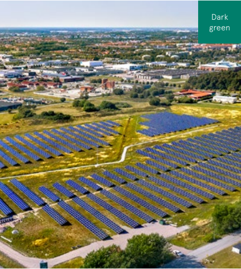
Solar park, Uppsala. The facility consists of 18,000 panels with a total area of around 30,000 square meters.
